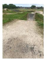
The BMX Track has many worn areas in the fine grit surface and is in need resurfacing.
